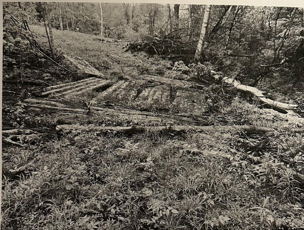
Photo 1: Timber Mat Crossing of Wetland
